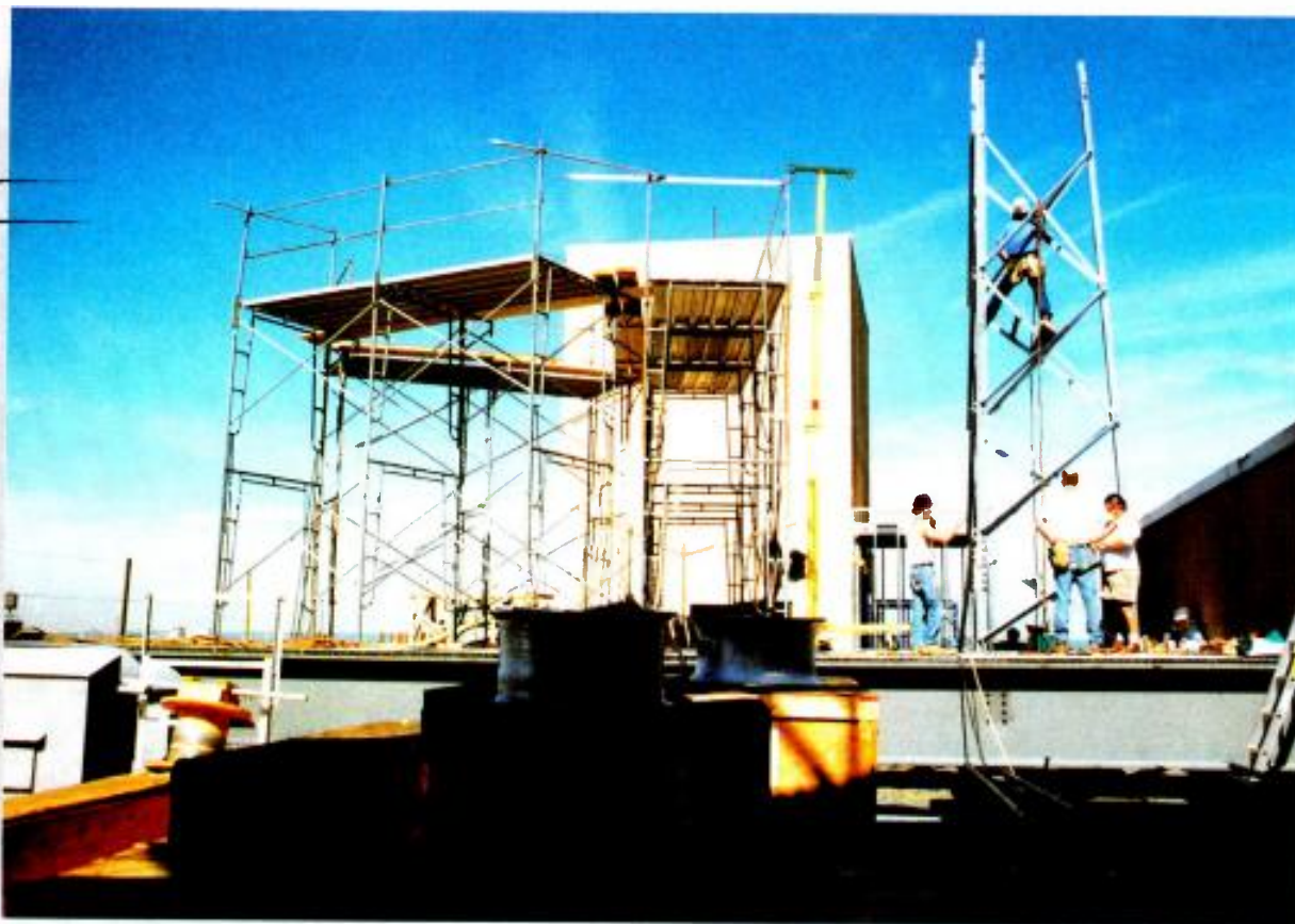
Rooftop RF support for 7.6m steerable and 7.3m fixed receive-only satellite antennas, assorted VSAT and DSS antennas, plus a 60-foot microwave tower.
